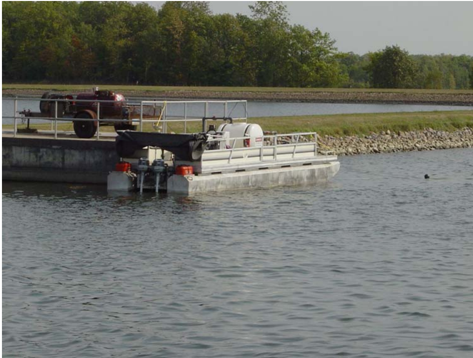
Figure 1 : Generator and Pump Trailer and Alum Application Boat at boat dock at Pond #3, Isle, MN. Isle Wastewater Treatment System has a boat equipped with a storage tank with chemical feed equipment and an outboard motor for alum applications. The alum is fed into the prop wash and mixed as a result of the action of the outboard (propeller driven) motor.
