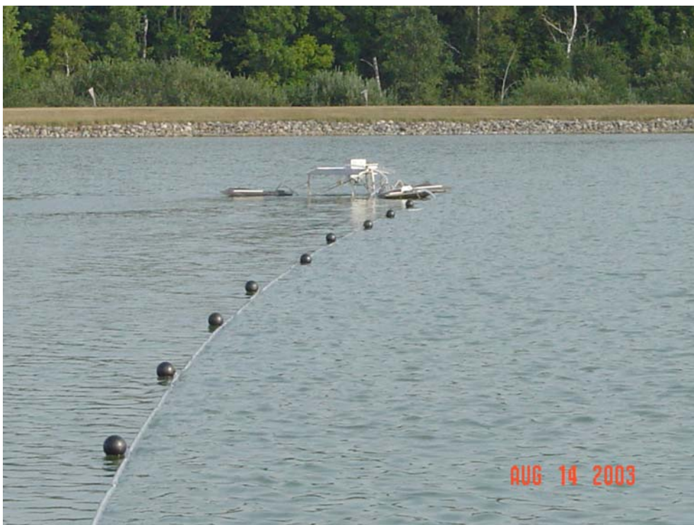
Figure 15 : The circulator at Test 3 at Isle. The floats support the discharge hose and 24-hour shore power cord from shore. Floats attached to the hose help suspend it in the water to prevent any disturbance of pond sediment. Alum has not yet been injected in this photo.
