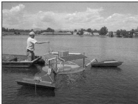
Mike Borsma of Pump Systems, Inc. installs the Solar Bee in Silver Lake.
