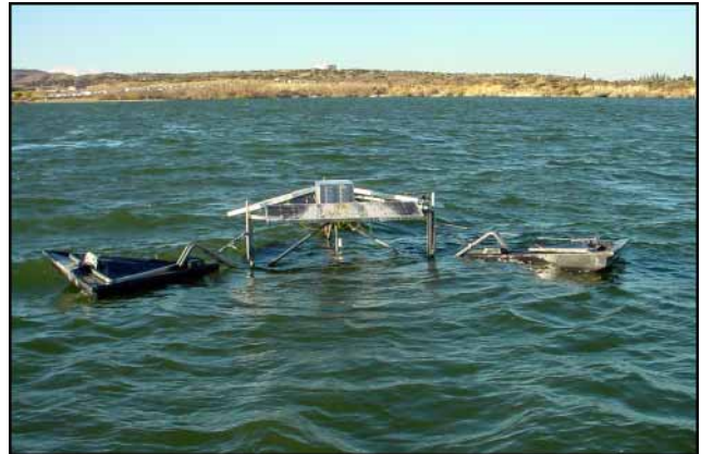
The Palmdale (California) Water District had been using up to 3,000 lbs. of copper sulfate powder per week to control algae growth in its 4,130 acre-ft. lake until it put in a SolarBee unit.
