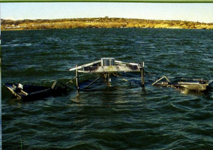
The Palmdale (Calif.) Water District had been using up to 3,000 lb of copper sulfate powder per week to control algae growth in its 4,130 ac-ft lake until it put in a Solar Bee unit.
