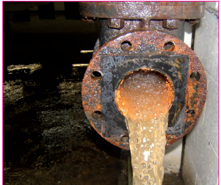
A typical building water meter replacement
